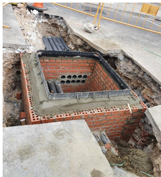
Figure 5: a renovated manhole in the city centre
