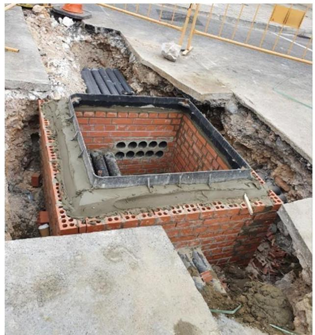
*Figure 5: a renovated manhole in the city centre*
